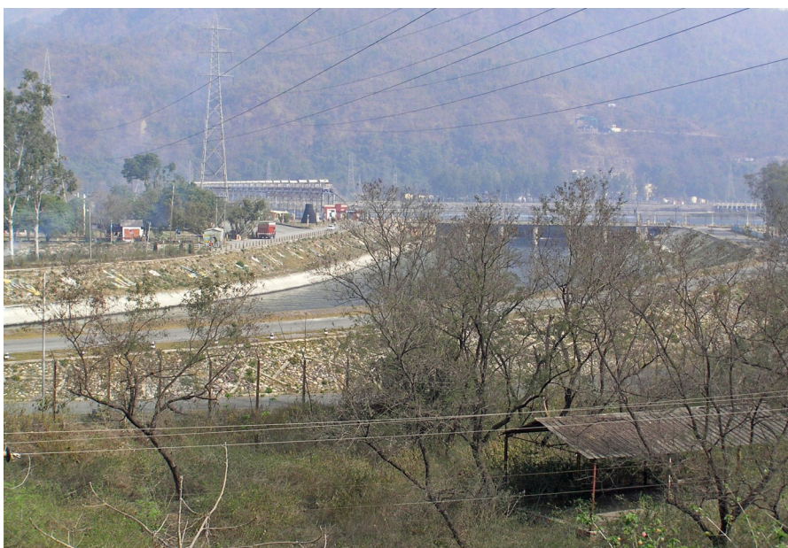
Canal off-taking from Hathnikund Barrage on the Yamuna River
